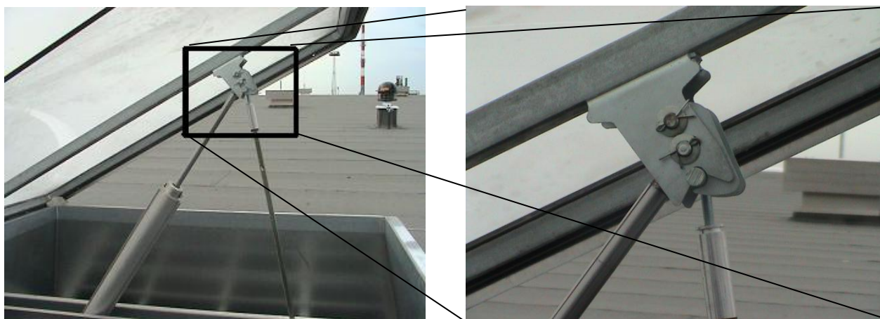
Fig. 24 Connection of the actuators with the hook lock.
